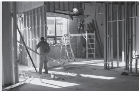
Pictured here is the employment benefits area currently under construction.
