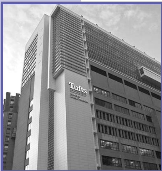
Top photo: Vertical expansion underway. Middle: New state-of-the art simulation lab. Bottom: Project completed. It's now a 15-story building.
